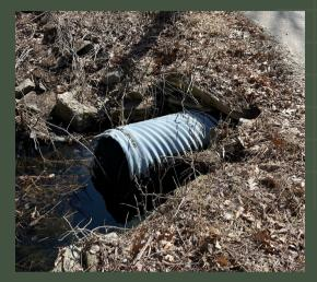
A good culvert lets the water continuously flow and without noticing the road being there. A bad culvert can restrict water, impact water quality, cause flooding, and/or create barriers to fish and other wildlife.
