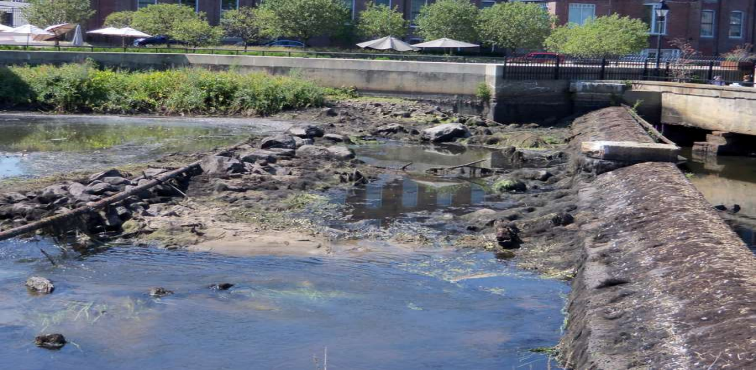
Case Study – Ipswich Mills Dam 33
